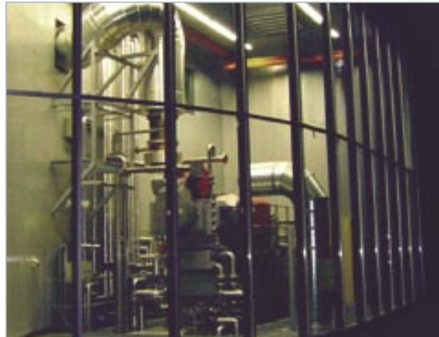
Fig. A2: Fritzens, Innsbruck/Austria Engine: 6L21/31, Output: 1 290 kW Fuel: Recycled frying fat
